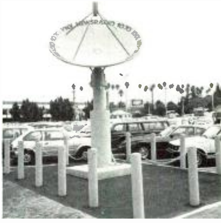
Since the CBS network has gone to satellite delivery of its program material, KNX has installed a 2.8 m Scientific-Atlanta antenna in its parking lot.
